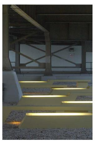
Internally-lit precast concrete bench
